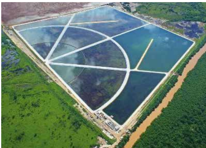
KMA Sewage Treatment, Jamaica
